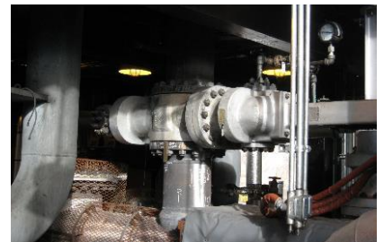
Slurry Isolation Valve with Emergency Shut Down (ESD) Actuation
